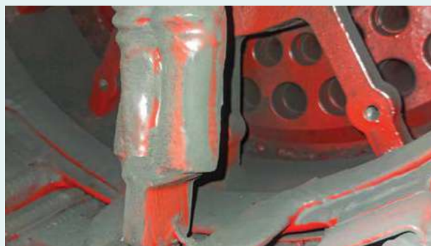
Carbon dust accumulation
